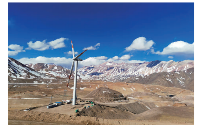
▲ Wind power generation by Veladero Gold Mine
