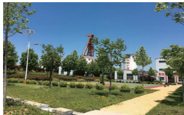
▲ Construction of green mines by Laixi Company
