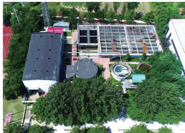
▲ Sewage treatment plant
