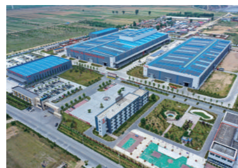
▲ Plant area of sdg heavy industry
