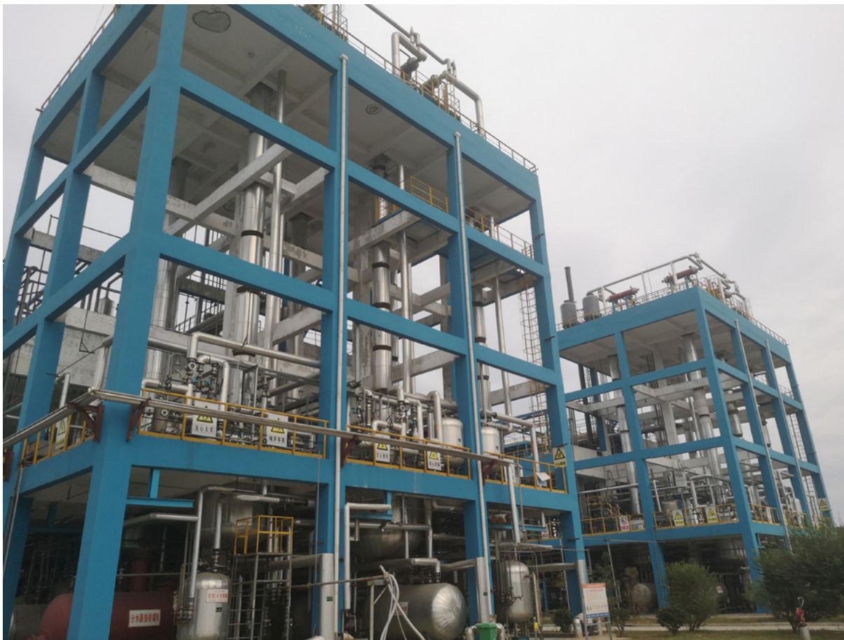
The Phase II of ethylene dichloride waste liquid treatment project
