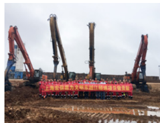
Participating in the construction of the first cross-river tunnel in Haikou
