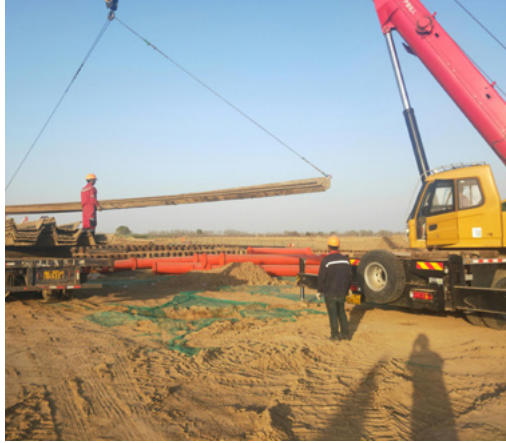
Participate in the Construction of Jingxiong Intercity Railway
