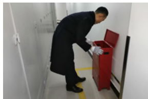
Regular Inspection of Fire Equipment
