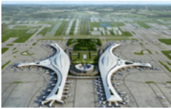
Participate in Scaffolding Project of ChengduTianfu International Airport
