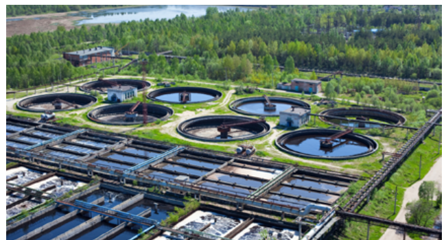
Sewage treatment plant
