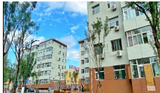
Photo of buildings after renovation
