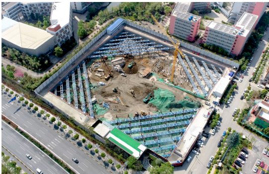
Undertaking the foundation pit supporting project of Yilai Business Center in Kunming
