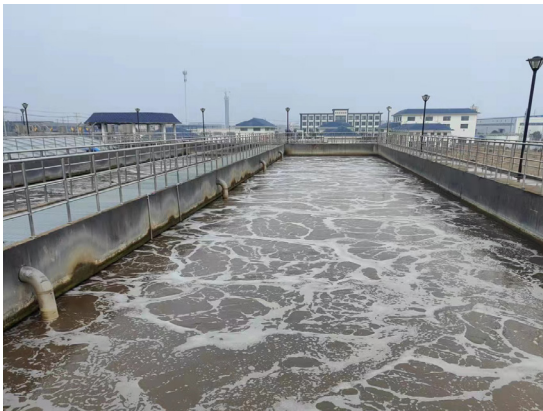
Photo of the sewage treatment plant
