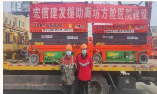
Supporting the construction of mobile cabin hospitals in Langfang
