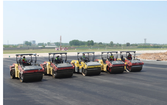
Participating in the construction of Zhengzhou Xinzheng International Airport (phase II)
