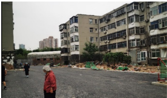
Photo of buildings before renovation
