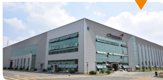
定建实景图 Real picture of Built-To-Suit workshop
