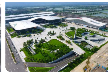
肇庆高铁东站 Zhaoqing East High-speed Rail Station
