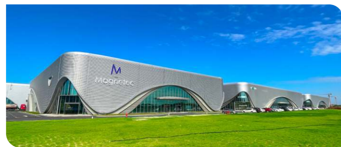
● P1单层厂房 P1 Single-storey Workshops
