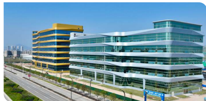
● P2多层厂房 P2 Multi-storey Workshops
