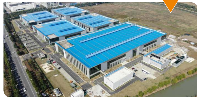
定建实景图 Real picture of Built-To-Suit workshop
